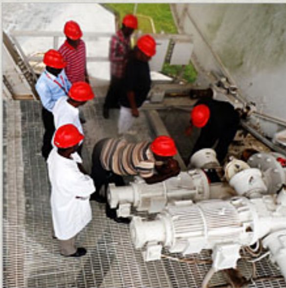
Conversion work on the dish in Ghana
