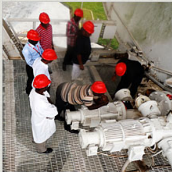
Conversion work on the dish in Ghana
